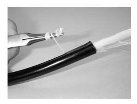
Figure 14 - Pull the ripcord through the inner jacket.
