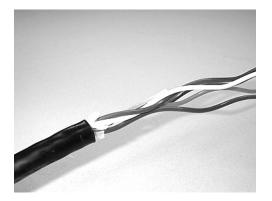
Figure 36 - Unwrap the buffer tubes.
