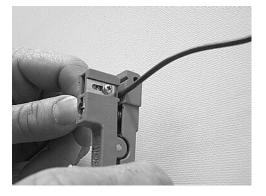
Figure 37 – Cut the buffer tubes to the required length.
