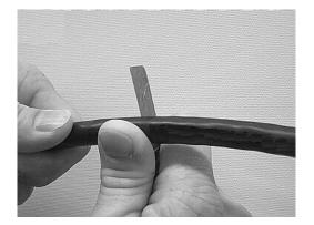
Figure 21 – Ring cut the cable jacket.
