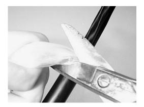
Figure 9 – Cut the dielectric strength members to the required length.
