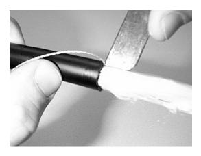
Figure 25 – Cut a starting slit adjacent to the ripcord.
