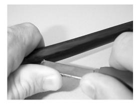
Figure 12 - Make a longitudinal cut at the end of the cable.
