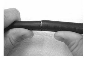
Figure 3 - Separate the cable sheath.
