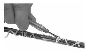
Figure 16 - Remove the binder threads and water blocking tape.
