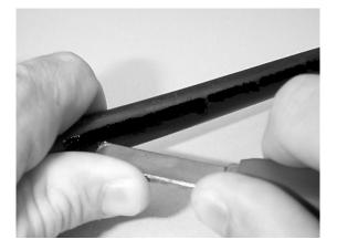
Figure 23 – Make a longitudinal cut at the end of cable jacket.
