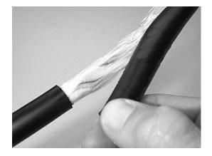
Figure 27 – Remove the cable sheath.
