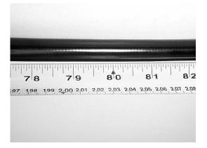
Figure 20 - Measure and mark the cable jacket for removal.
